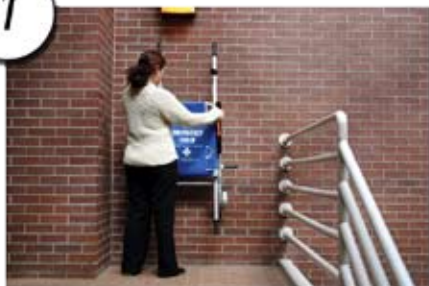
The chair is easily accessible as it is wall mounted near each stairwell for use in emergencies.
